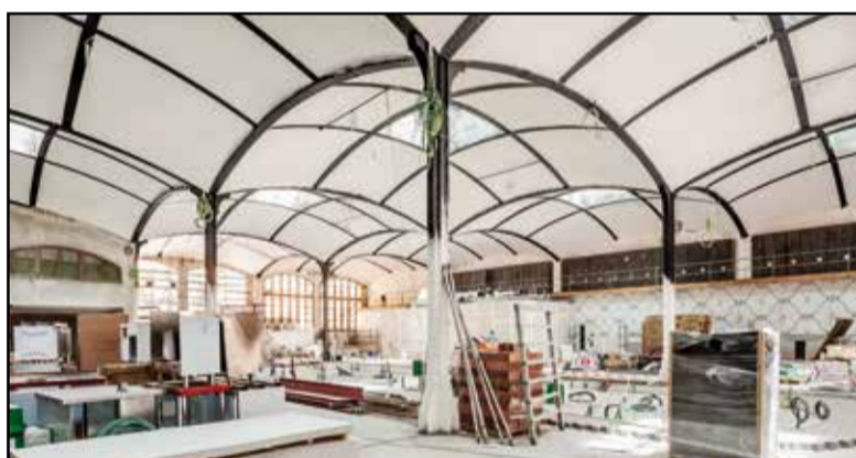
El Nacional before being refurbished. / El Nacional abans de la reforma.
